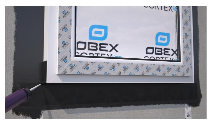
Apply a small section of OBEX CORTEX 0771FR Class B Paste Adhesive to the corner area as shown. (both sides of the window frame)
