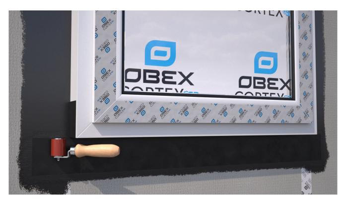
Bond the second half of the membrane into position and firmly roll with a roller.
