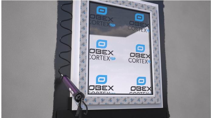
Apply OBEX CORTEX 0769 Paste Adhesive to the sides of the frame and substrate.
