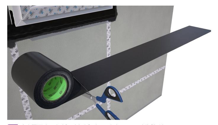
Cut the EPDM Membrane to length. Ensure the length of membrane extends at least 100mm past each side of the window.
