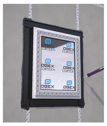
Apply a bead of OBEX CORTEX 0769 Paste Adhesive around the perimeter and over any joints/overlaps.
