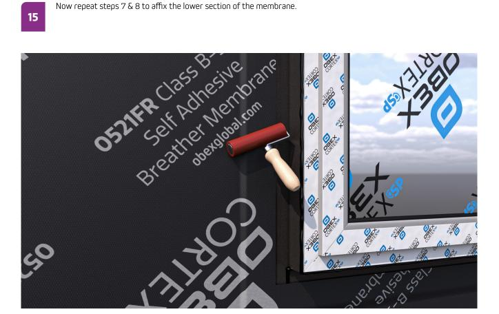
Use the roller to ensure that the edge of the membrane is bonded firmly onto the ISM around the window.
