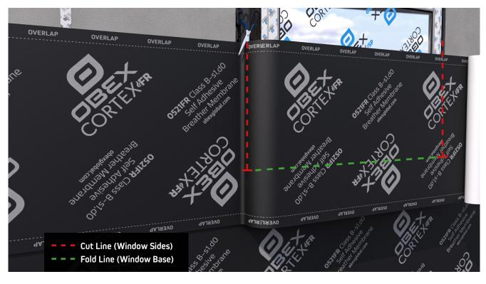
Only cut down as far as the bottom corner of the window, unroll the membrane across the window and repeat the same length cut on the opposite side.
