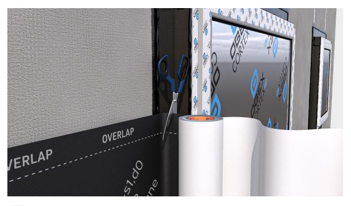
Cut the membrane to length, allowing 100mm to overlap the ISM (Interface Sealing Membrane) around the window. Use Membrane Shears rather than a knife, to ensure the ISM is not damaged.
