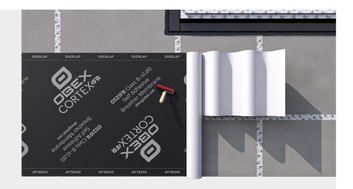
Continue to remove the top release liner, whilst simultaneously applying the membrane to the substrate. Use the roller to ensure it is firmly adhered.
