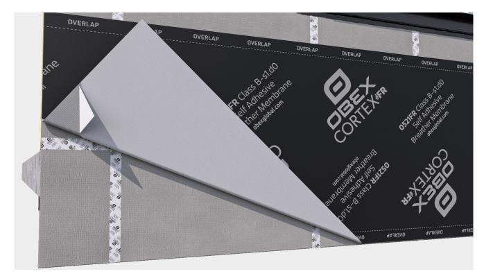
Now peel away the lower section of the release liner and affix the membrane to the substrate as before.
